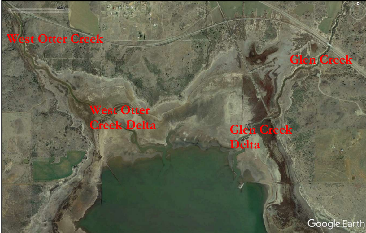
Figure 11. Google Earth imagery from 2014 showing exposed deltas on upper end of Tom Steed Reservoir from the two main tributaries.
