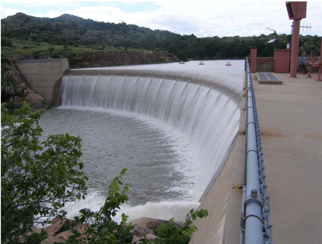
Figure 9. Mountain Park Dam and operating spillway (Ferrari, 2010).
